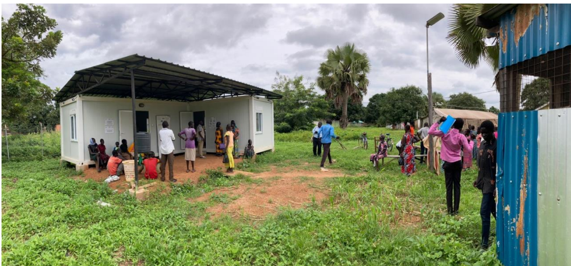
The new epilepsy clinic, built by the NSAlliance in May 2022
