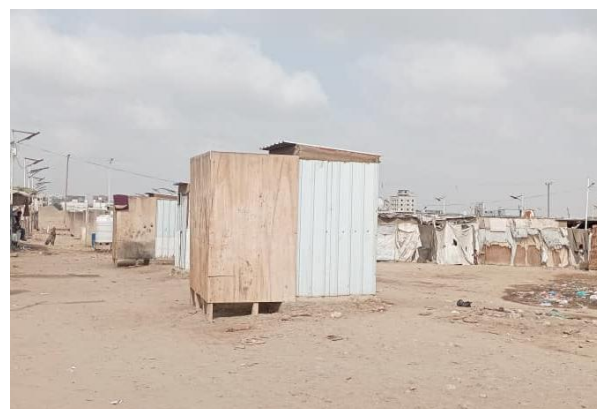
Emergency Latrines for Females Installed in Al-Ribat IDP Camp as Part of WASH Response May, 2025
