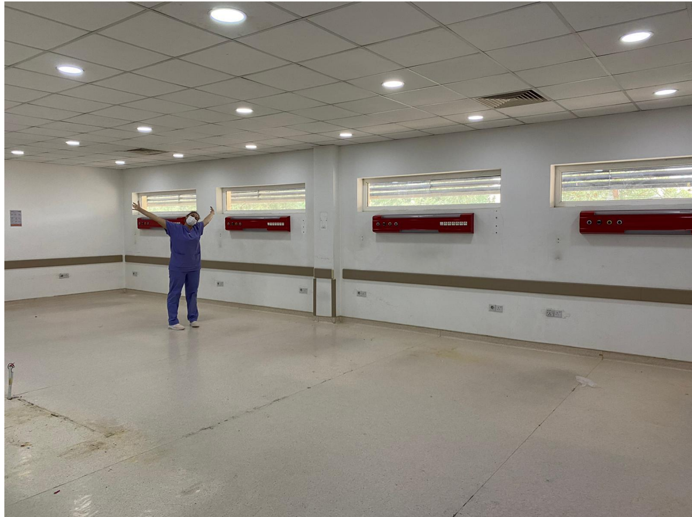
Expansion of the Pediatric Neonatal Intensive Care Unit at Hevi Pediatric Hospital.
