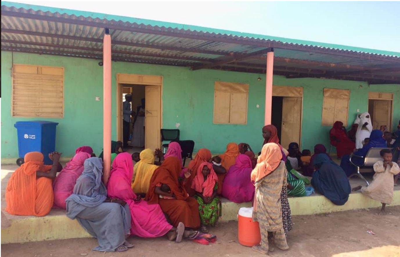
BELOW: Rehabilitation of 3 health centers in Um Alqura, Issa Al Haj and Hadalia, including installation and activation of water points and rehabilitation of latrines.
