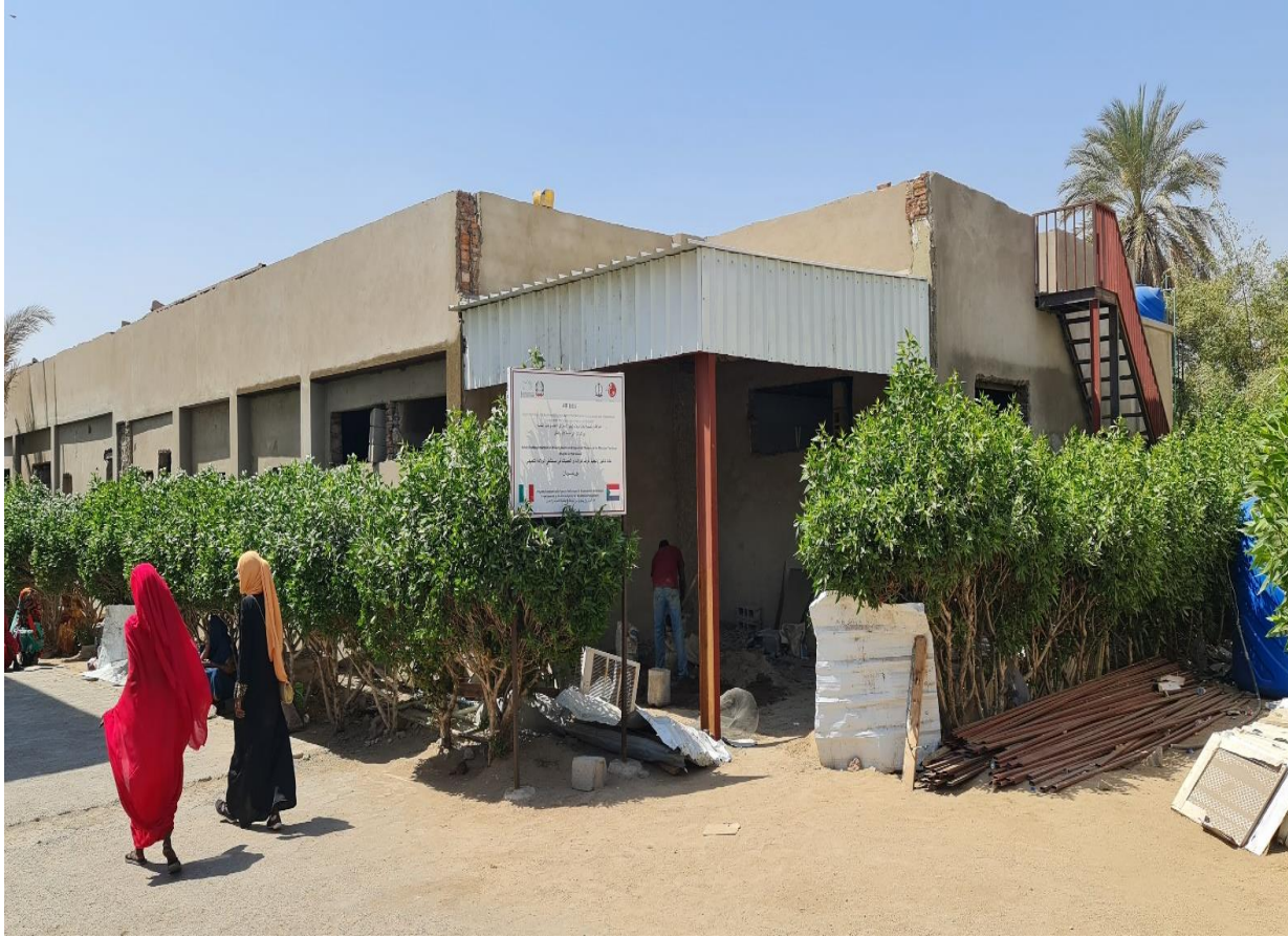
Rehabilitation and expansion of the operating theater and delivery rooms of the Maternity Hospital in Port Sudan
