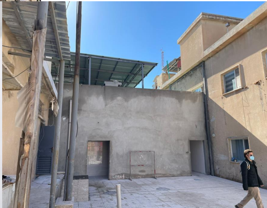
TOP & LEFT: Exterior of the new operating block in March 2021
