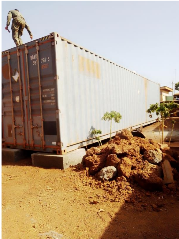
Arrival of the container to Wau Hospital with the equipment for the rehabilitation of the hospital's electrical panel
