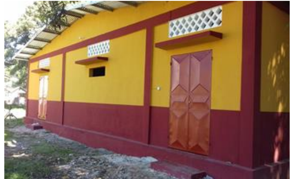
Exterior of the dispensary
